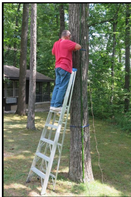
KC9UR Installing the Horizontal Antenna
